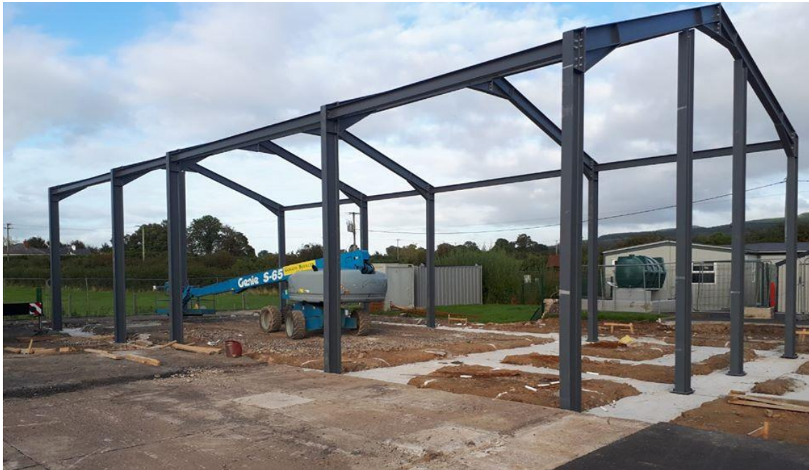
School Hall Initial Building Phase
