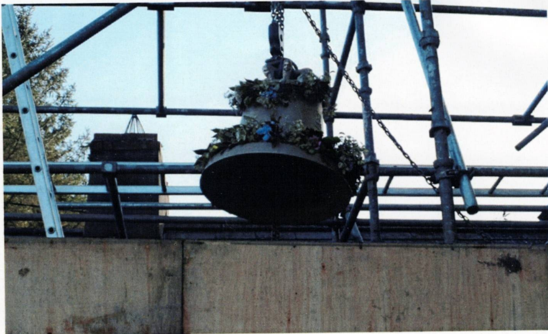
The Bell being raised into the Belfry
